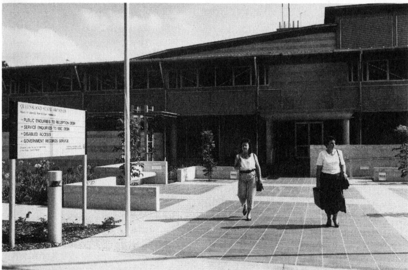
The new premises of the Queensland State Archives at Runcorn. Public Entrance.
