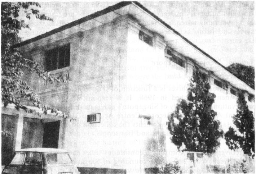
Former Singapore National Archives Building at Fort Canning.
