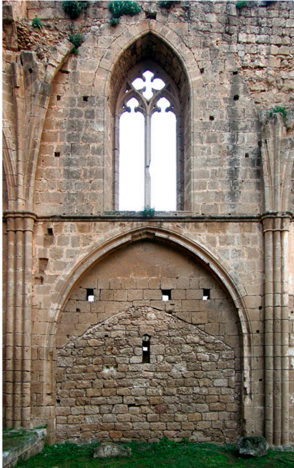
Figure 3. Southern wall (4th bay) of St George incorporating northern wall of the older Hagios Epiphanius. Photograph by Thomas Kaffenberger.
