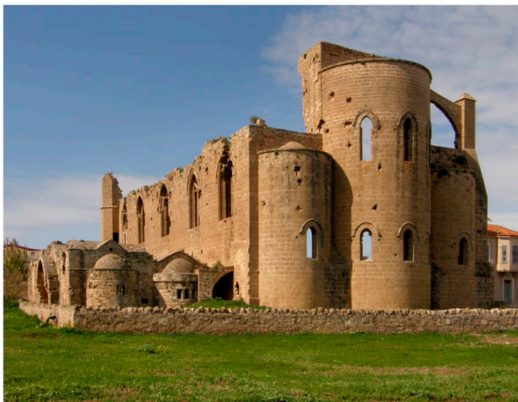
Figure 2. Hagios Georgios (right larger structure) and Hagios Epiphanios (left smaller structure), south-eastern facades. Photograph by Thomas Kaffenberger.
