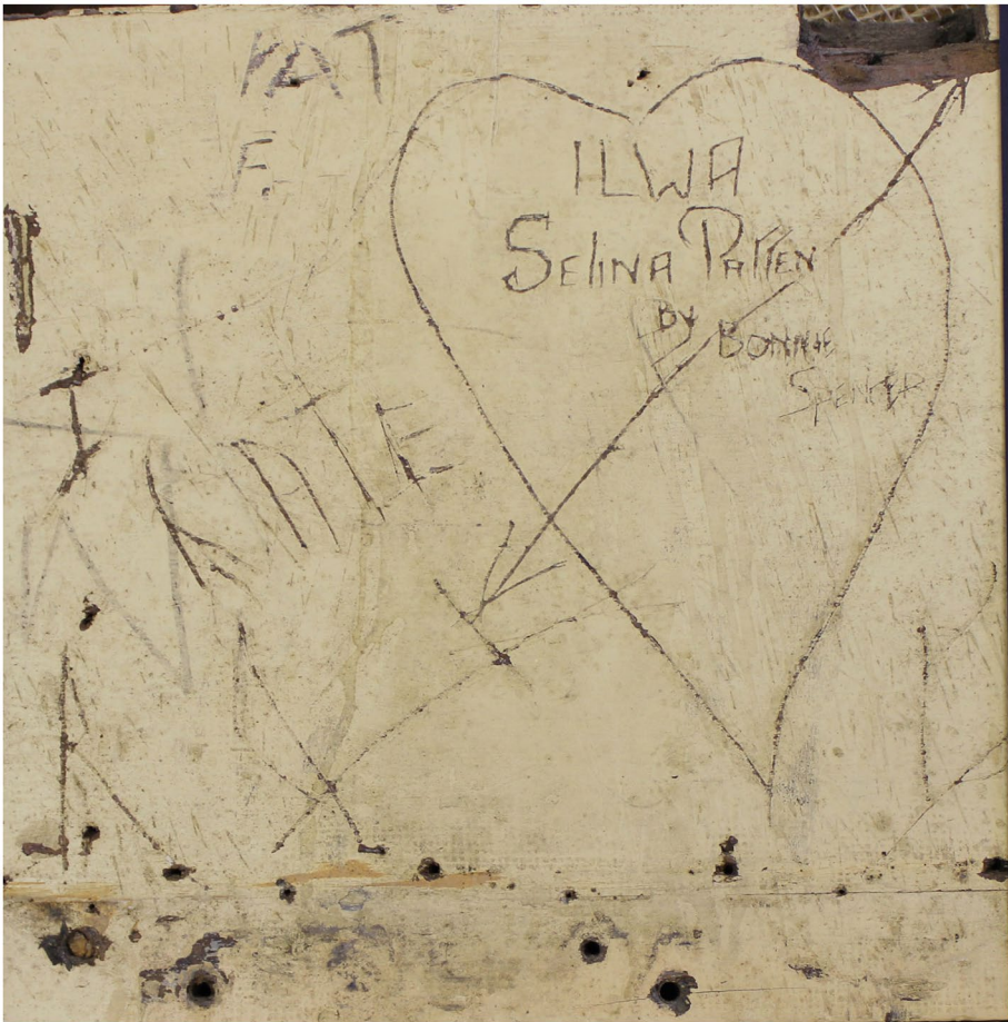
Figure 5. Graffiti on segregation room door, Parramatta Girls Home; photo Bonney Djuric.
